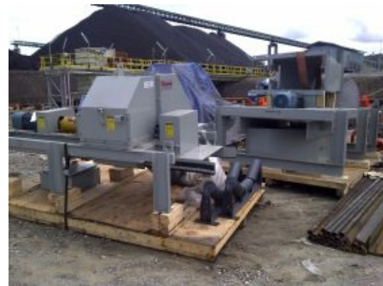
Commissioning and Installation
